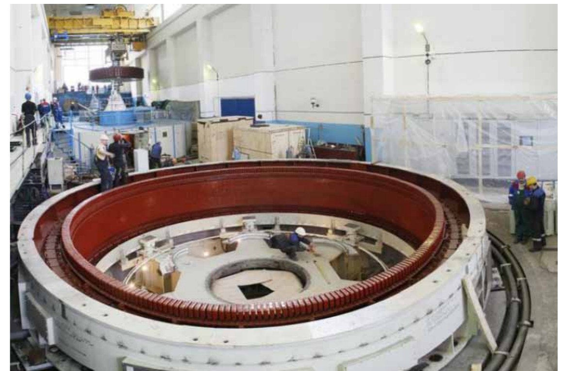
Fig. 26. Installation of a rotor of a Hydropower Unit at Lesogorskaya HPP
