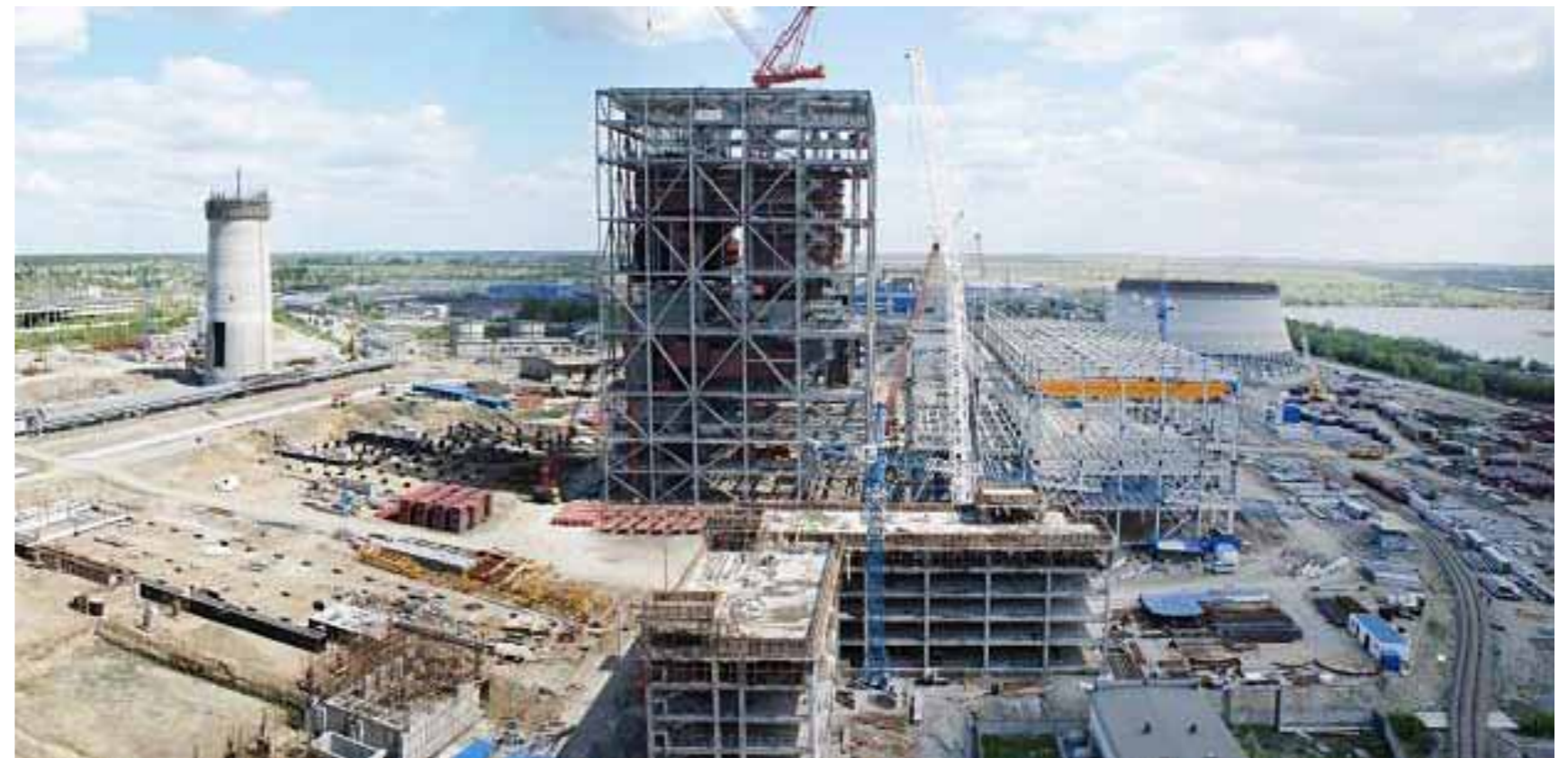
Fig. 33. Construction of a new coal dust generation unit at Troitskaya GRES
