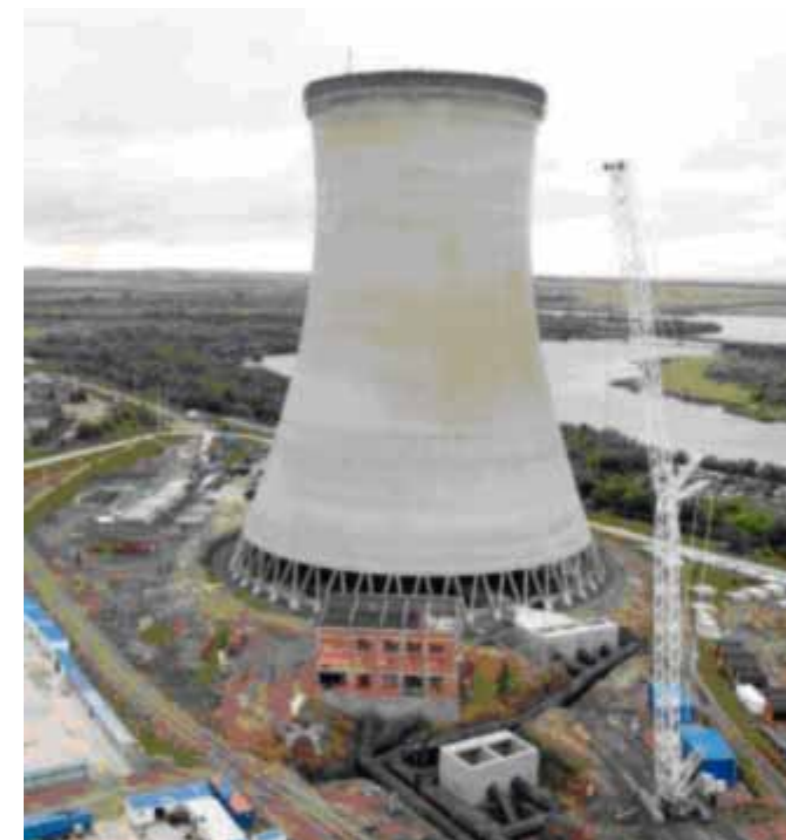
Fig. 23. Concreting of a cooling tower building at Troitskaya GRES
