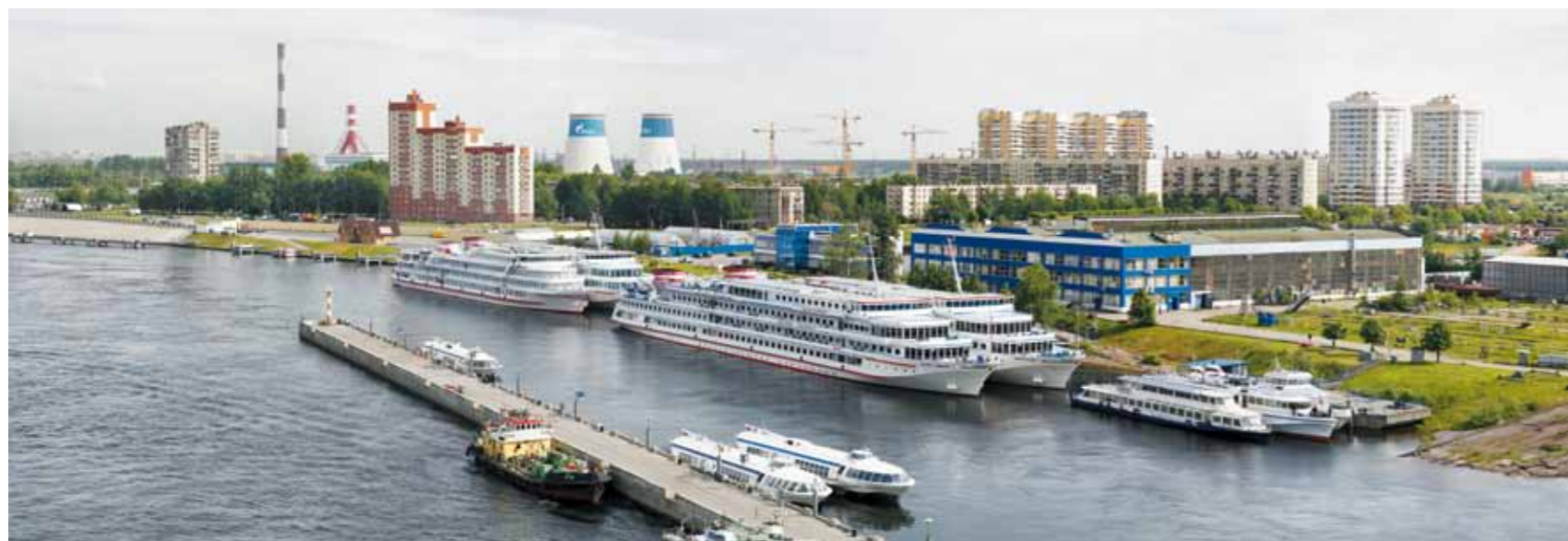
Fig. 10. Pravoberezhnaya CHP. Nevsky Branch
