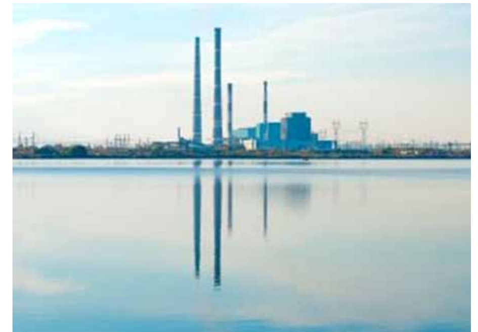
Fig. 48. Ryazanskaya GRES at Novomichurinskoye Reservoir
