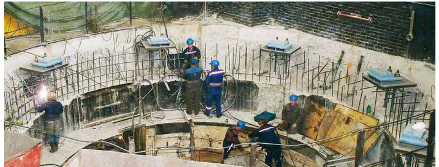
Fig. 25. Installation of Hydropower Unit No. 3 at Lesogorskaya HPP
