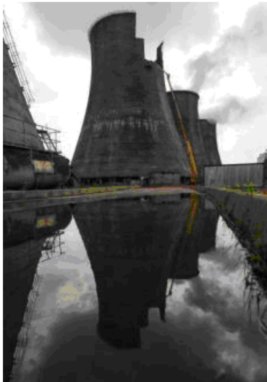
Fig. 21. TPP-16: Disassembly of Cooling Tower No. 2
